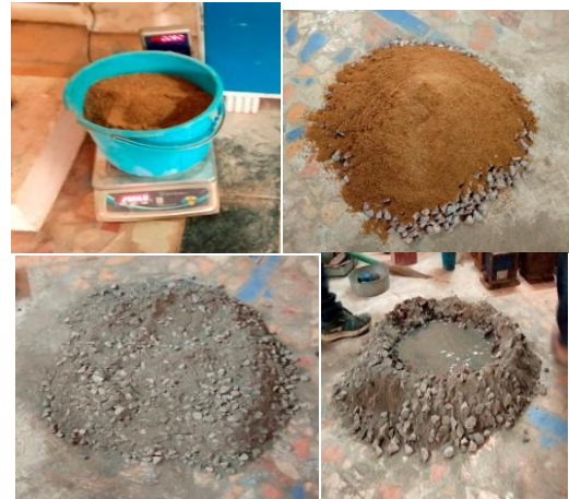
Fig.-2 Weight batching and mix of concrete
